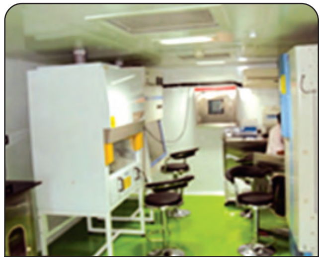
BSL-3 upgrades at BPHRC, Hyderabad.
